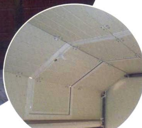
Peatonal interior abriendo
